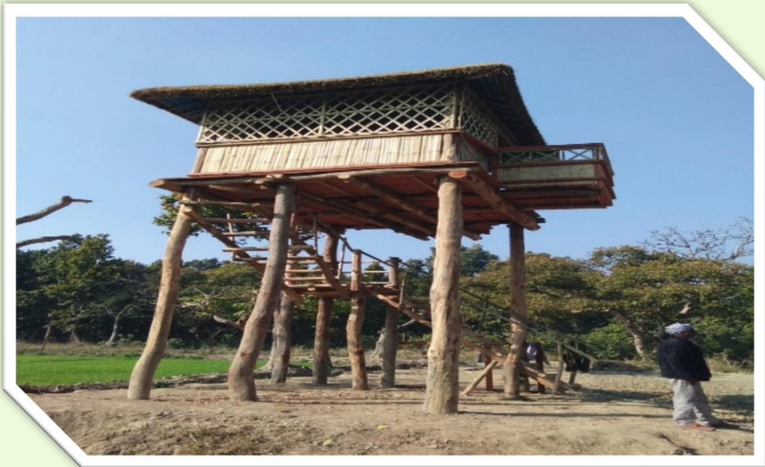
Pilibhit Tiger Reserve, Construction of Watch Tower
